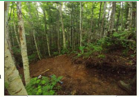
A trail under construction
