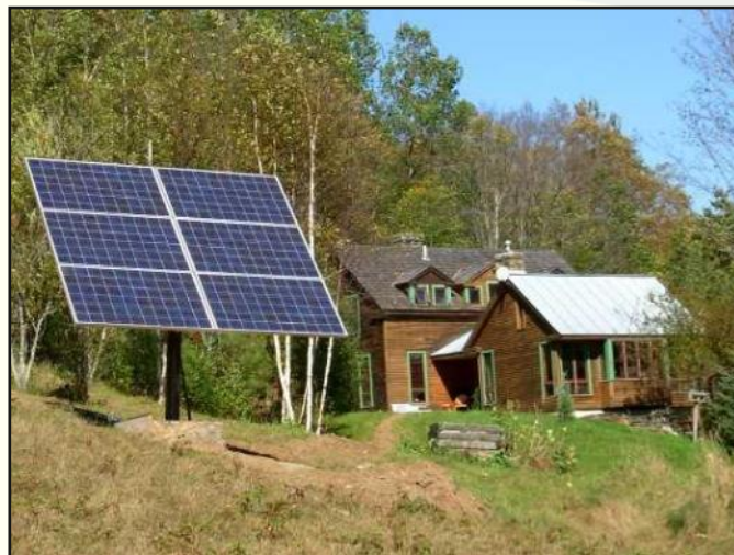
A ground-mounted solar panel system
